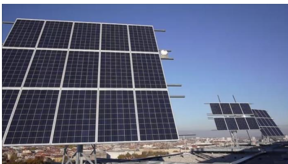
Photovoltaic power plant
